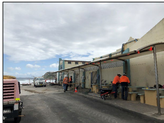
Photo 8 – View of the rear the existing amenity buildings facing southwest.
