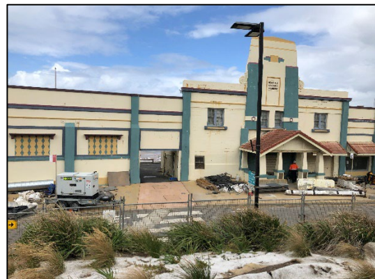
Photo 4 – View of the existing Ocean Bath facilities facing east.
