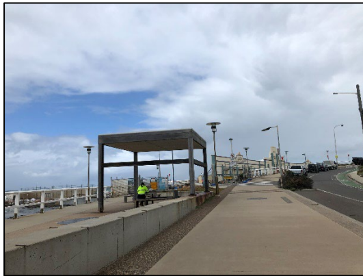
Photo 1 – View of the works area along Shortland Esplanade facing south.
