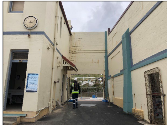
Photo 6 – View between the existing amenity buildings facing northwest.
