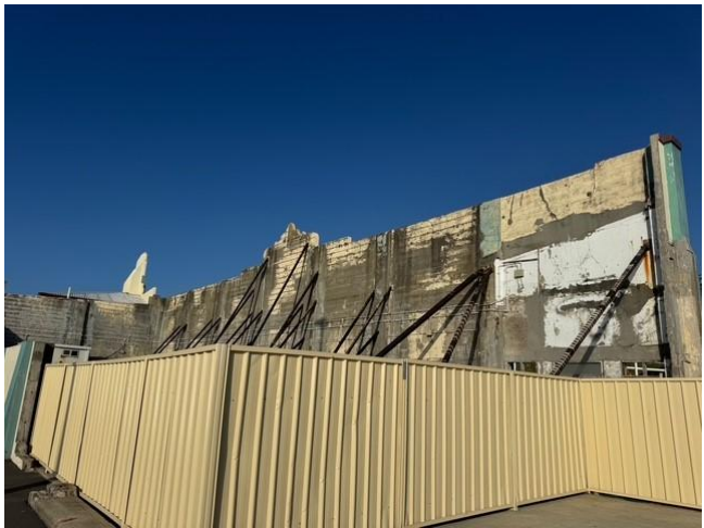
Picture 4 View of the north pavilion which currently only includes a façade towards the car park.
